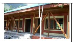
Retrofitting completed bracings between columns
