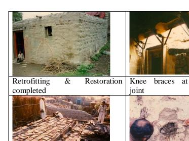
Upper Wall removed for band installation & Roof deck opened for repairs
