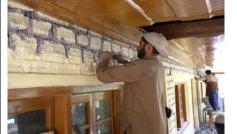
Installation of WWM for Lintle level Seismic Belt
